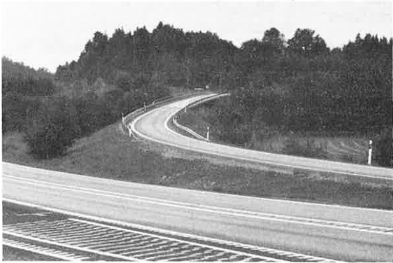
Figure 5.3 The westerly view of the exit ramp at Bratteröd test site.
